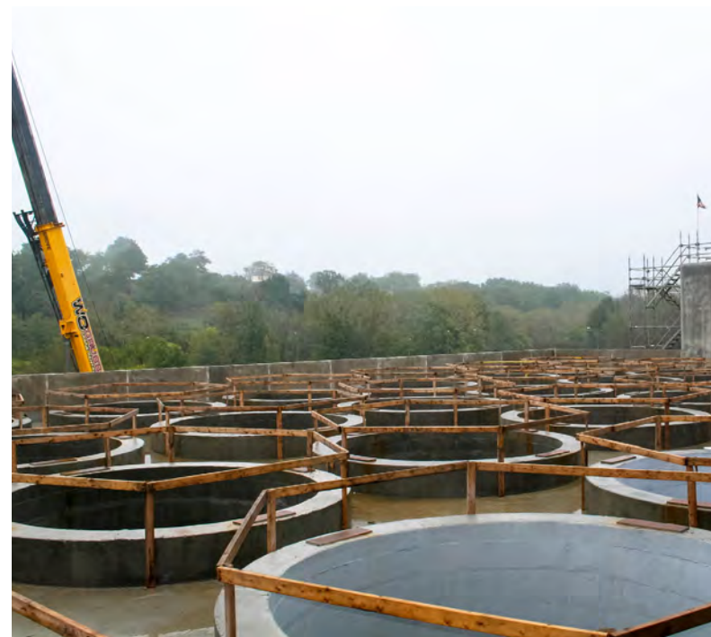
The five foot deep elevated cast-in-place concrete tank farm structure was designed to support 40 fermentation and bright tanks that support the annual production of 600,000 barrels per year.
