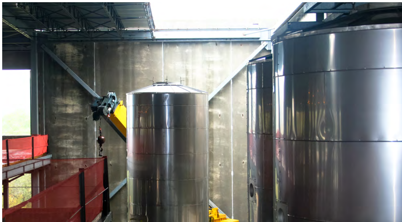
The elevated brew house mezzanine was designed with coordinated slab penetrations in the structural steel to accommodate all of the brewing equipment, including the lauter tun at over 25 feet in diameter. The roof structure was designed as a panelized system for removal of the roof assembly to allow for placement of water tanks, smaller fermentation vessels, and future equipment needs.
