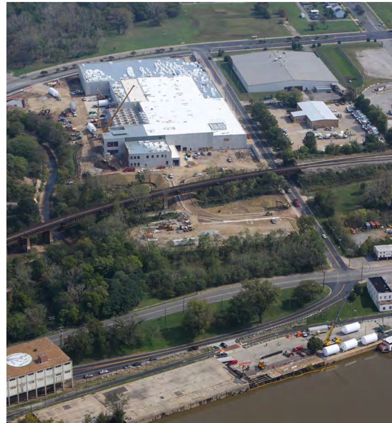
The project site consisted of 14.5 acres of developed site that includes 2 parking lots for 276 cars, and material receiving and distribution docks. The property was bisected by Gillies Creek and the CSX train tracks. 220 feet of reclaimed bridge will connect the parking to the front entry across Gillies Creek.
